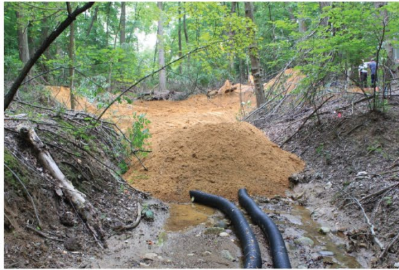
INSTALLATION CONDITION (DEWATERING PIPES)
