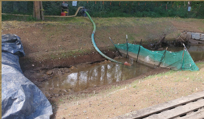
Left: Sandbag Diversion and fish exclusion netting
