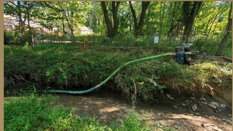
Right: Stream Diversion Pump and Discharge Hose
