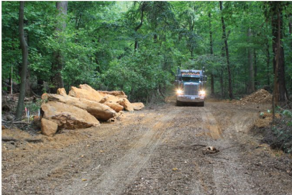
INSTALLATION CONDITION (DELIVERY OF MATERIALS)
