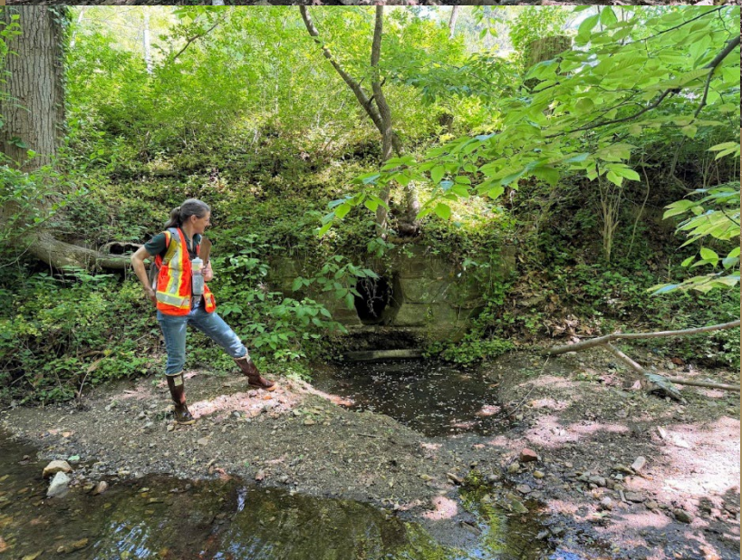
Four images showing how active streambank erosion has damaged existing storm drain outfall headwalls and aprons causing infrastructure instability.
