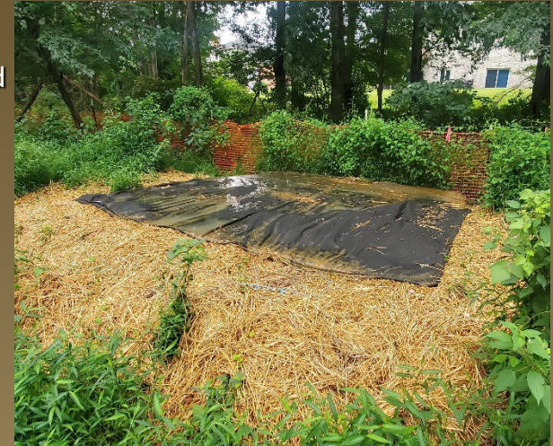
Right: Dewatering Device (filter bag)
