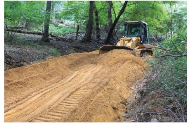
INSTALLATION CONDITION (FILLING CHANNEL WITH SAND AND GRADING ACCESS ROAD)
