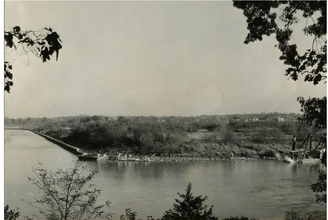
C. 1938 photo seawall construction (Living Classrooms, https://www.kingmanisland.com/ )
