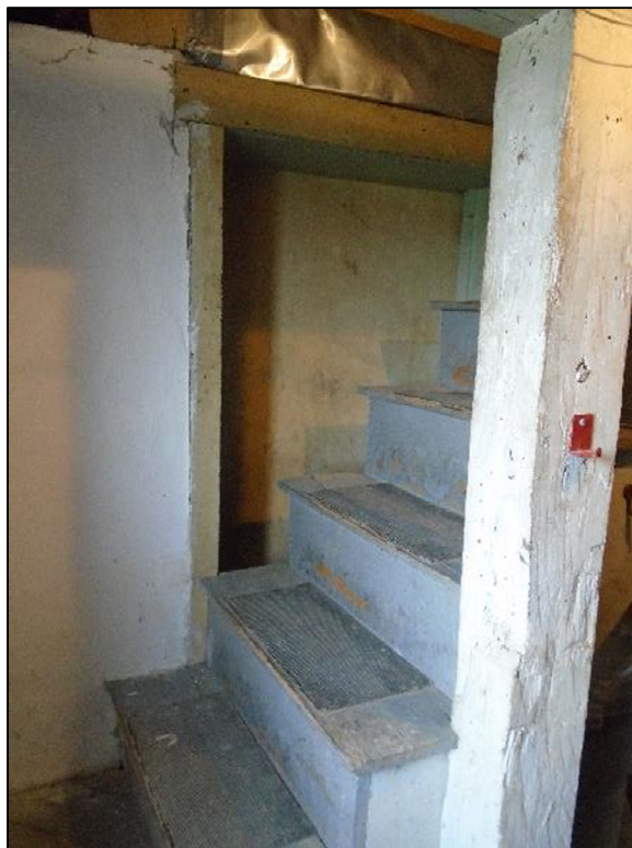
Photograph 19 – Original cellar door blocked by current basement stairs; looking northwest.
