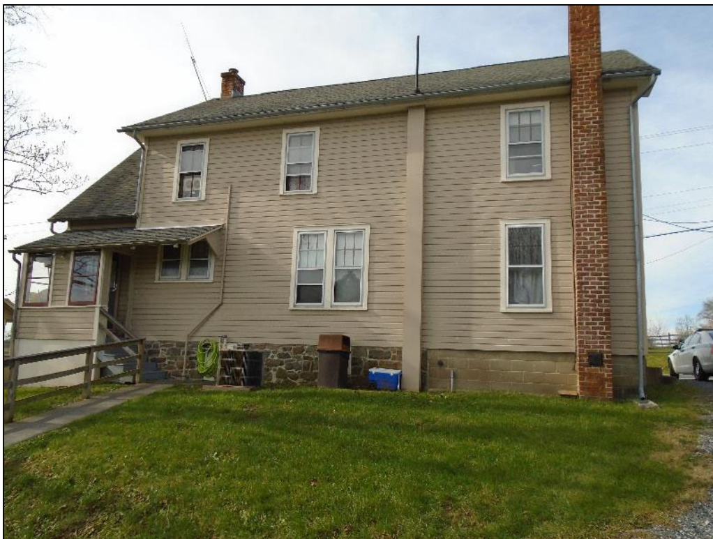
Photograph 3 – Rear (east elevation) of the dwelling looking west.
