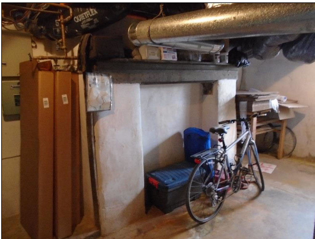
Photograph 18 – Infilled fireplace in basement, looking southwest.
