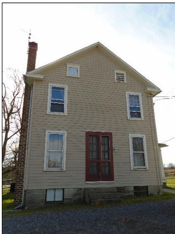
Photograph 2 – Side (north elevation) of the dwelling; looking south.
