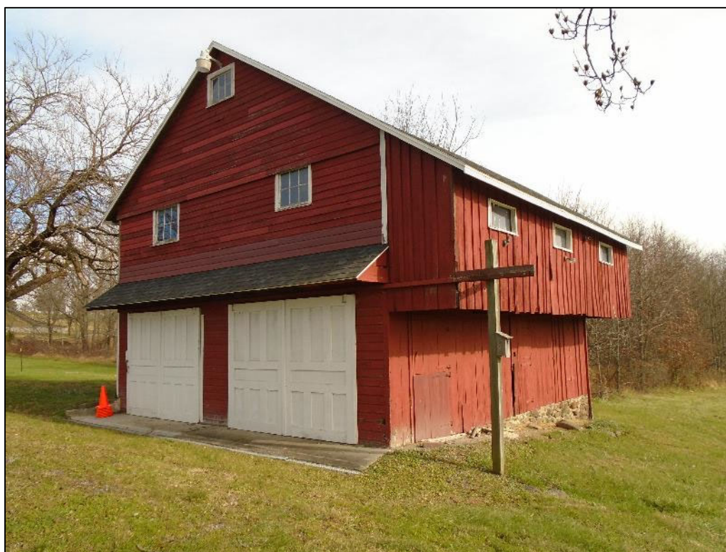
Photograph 20 – Façade (west elevation) of carriage house and shed; looking northeast.
