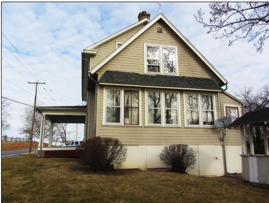
Photograph 5 – Side (south elevation) of the dwelling; looking north.
