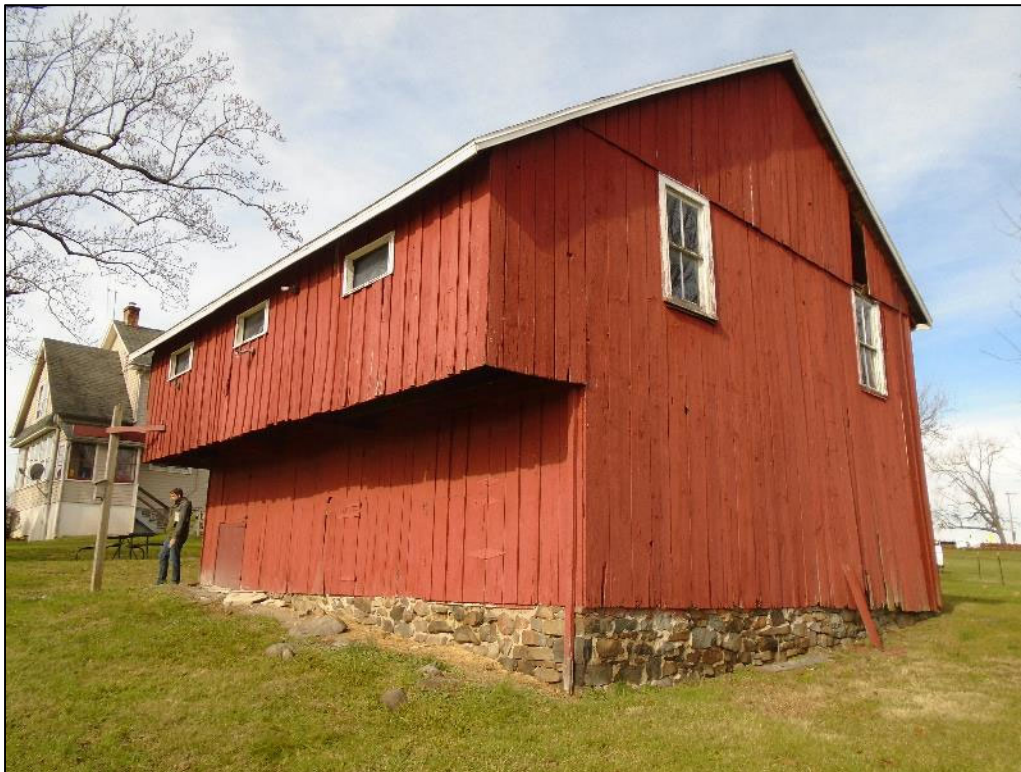
Photograph 21 – Side (south elevation) and rear (east elevation) of carriage house and shed; looking northwest.
