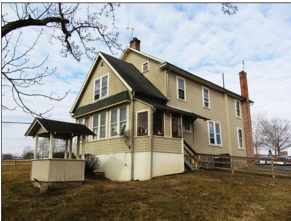
Photograph 4 – Rear (east elevation) and side (south elevation) of the dwelling; looking northwest.
