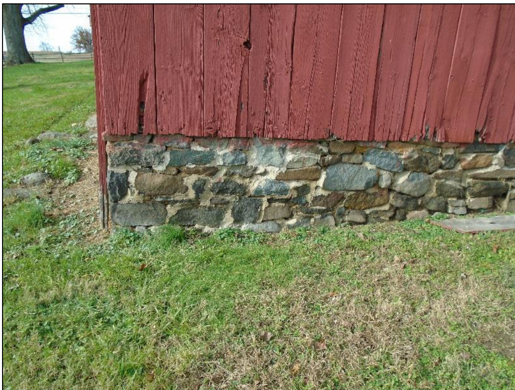
Photograph 22 – Detail of foundation on carriage house and shed.
