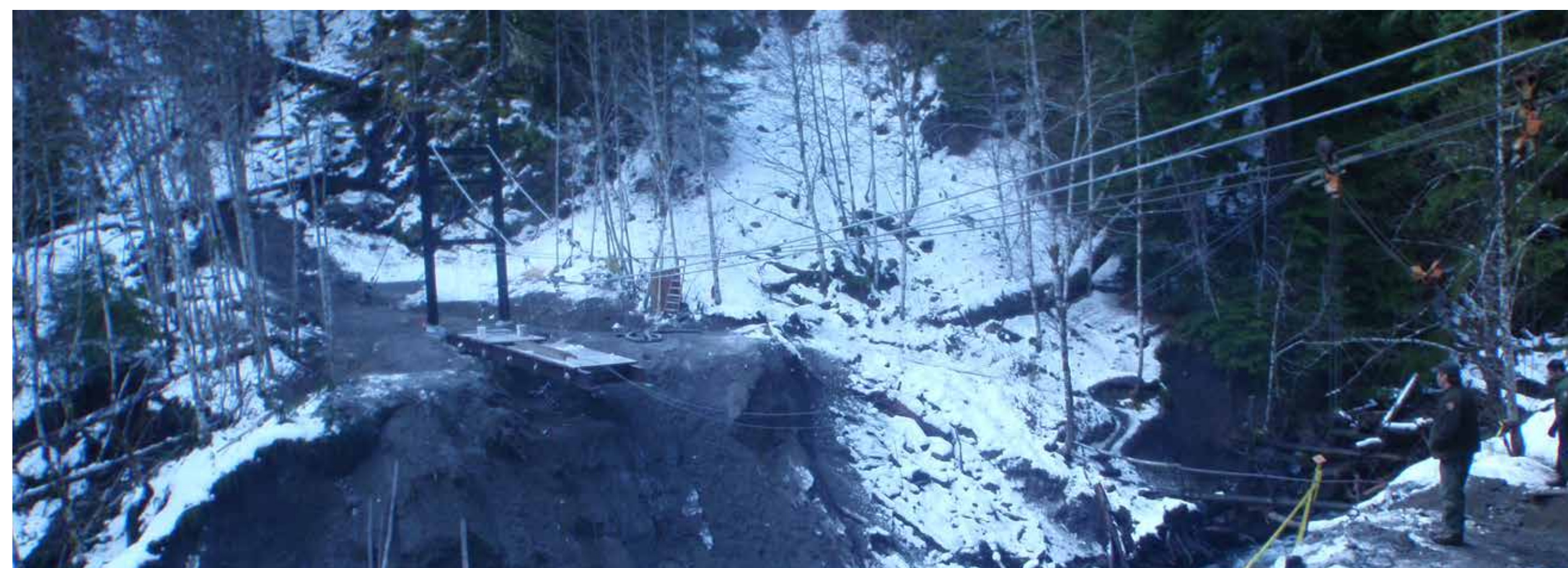
Cables hung, deck system being installed using the highline (In Progress)
