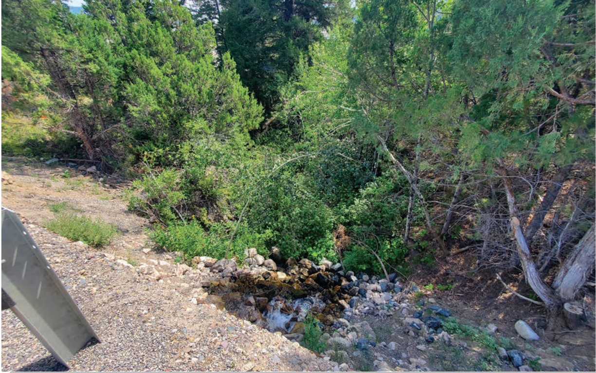
GAMA006s_92_pp – GAMA006s and Slide Lake tributary. View is to the northeast.
