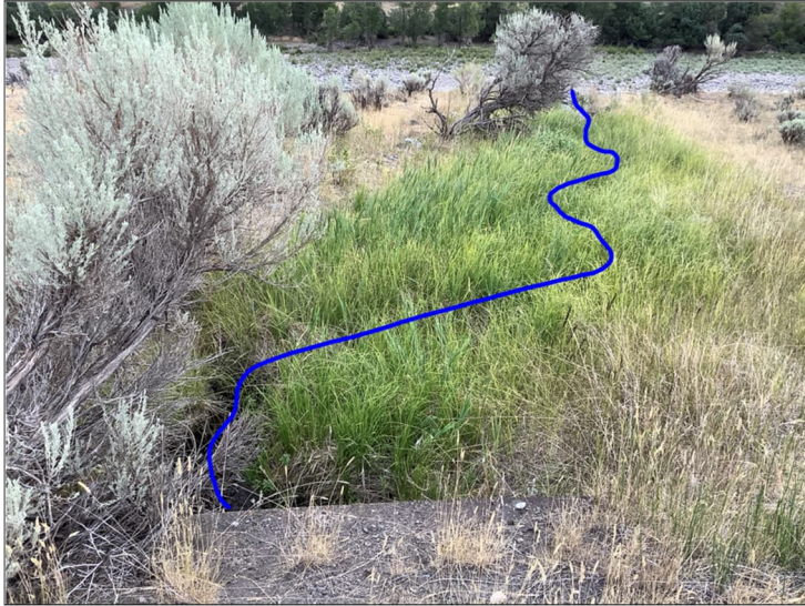
Photo 4. View to the north of Landslide Creek (blue line) flowing from the existing culvert towards the Yellowstone River. Proposed restoration activities would include replacing the culvert with a pedestrian bridge and enhancing the existing fringe wetlands with shrub plantings.
