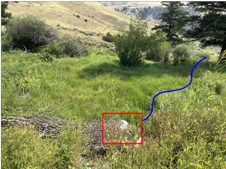
Photo 7. View to the northeast (downslope) of the Old Gardiner Road restoration site. The photo shows the existing culvert outlet (red square), stream (blue line), and wetland (foreground).
