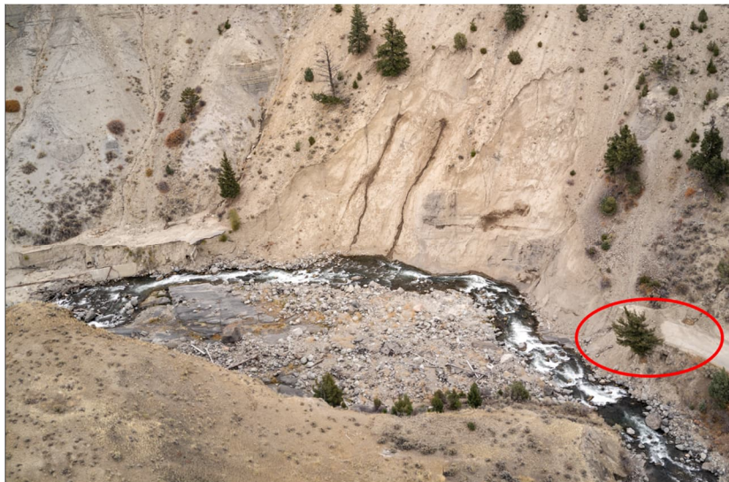
Photo 9. Overhead view of Gardner River Canyon (source: NPS). Bank stabilization (red circle) would maintain the integrity of remaining road elements converted to pedestrian trails.
