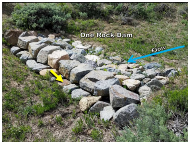
Photo 6. Example of Zeedyk structure (Maestas et al. 2018).
