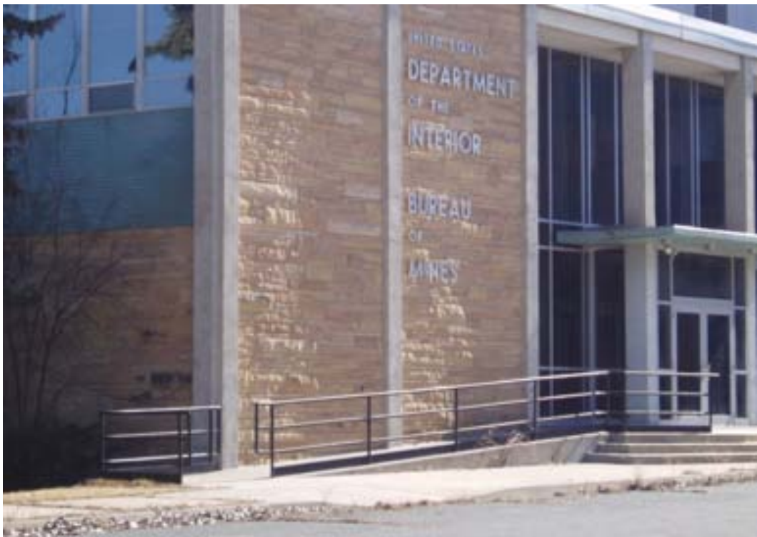
FIGURE 9. CLOSE-UP OF BUILDING 1 WITH VISIBLE BLUE, GLAZED BRICK AND LIMESTONE VENEER
