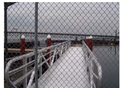
Gated entrance to the Riis Landing ferry dock
