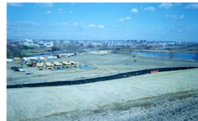
Administrative area during landfill capping
