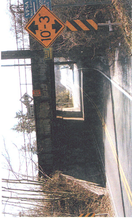
Photo 5: Looking east at the Pawlings Rd. underpass and the Norfolk & Southern railroad bridge where the substandard 10'-3" clearance limits use of the road by larger trucks, forcing them onto other roads such as PA 23 through the park.
