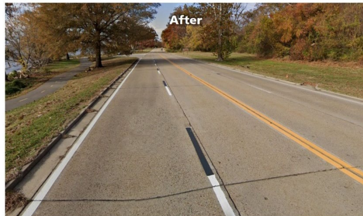
Contrast Pavement Markings
