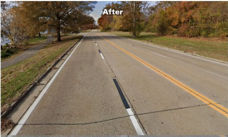
Contrast Pavement Markings
