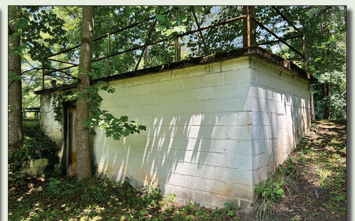
Camp Brookside Pool Chemical Treatment Plant
