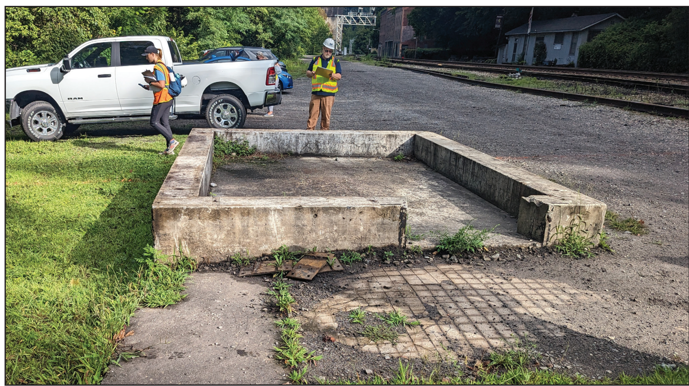
Foundation remains of the original location of the Thurmond Ice House. A similar approach may be taken for the structures in this project.
