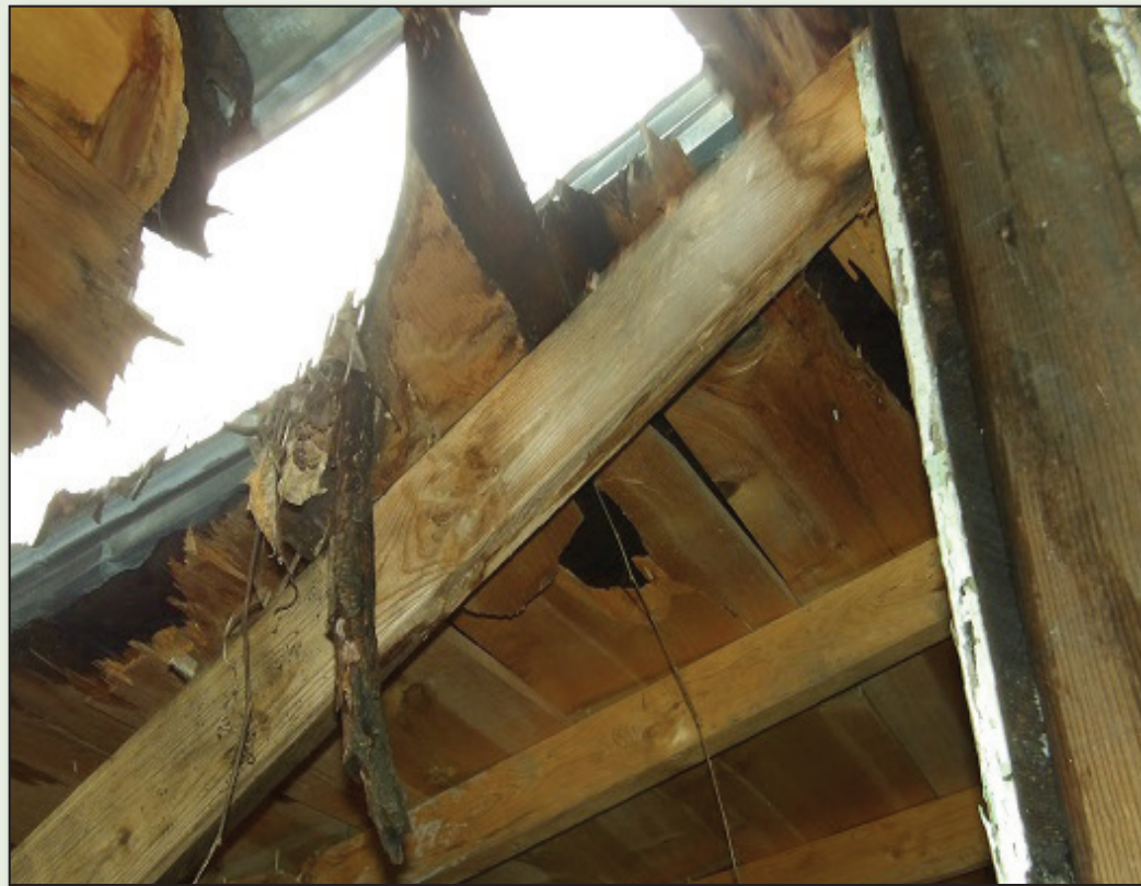
⑨ Erskine Pugh Rental House (interior)
