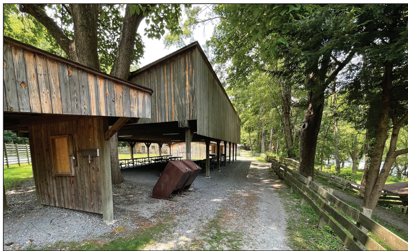
Picnic shelters at Dun Glen constructed and used by Wildwater Expeditions, Inc.
