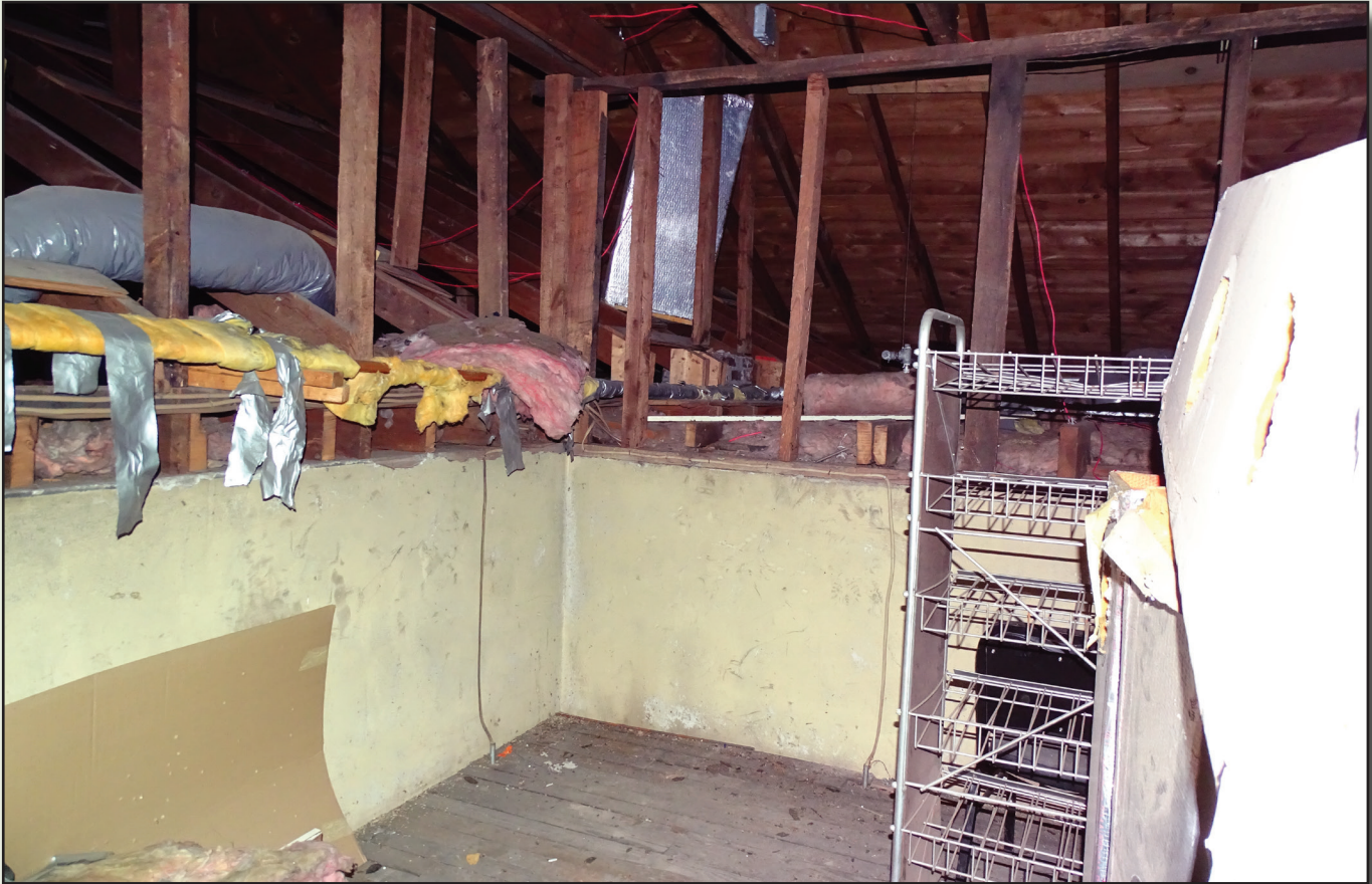
14 Dun Glen Building (interior)
