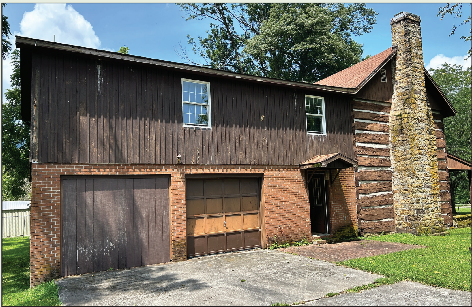
20 Vallandigham House Addition
