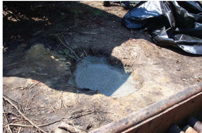
Well with plug in place.
