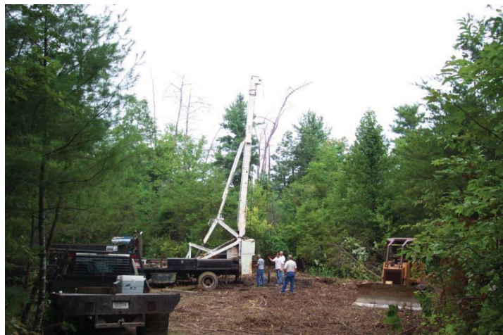
Pulling rigs used during well reclamation activities.
