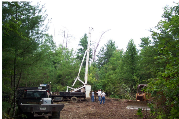
Pulling rigs used during well reclamation activities.
