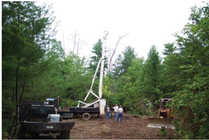
Pulling rigs used during well reclamation activities.
