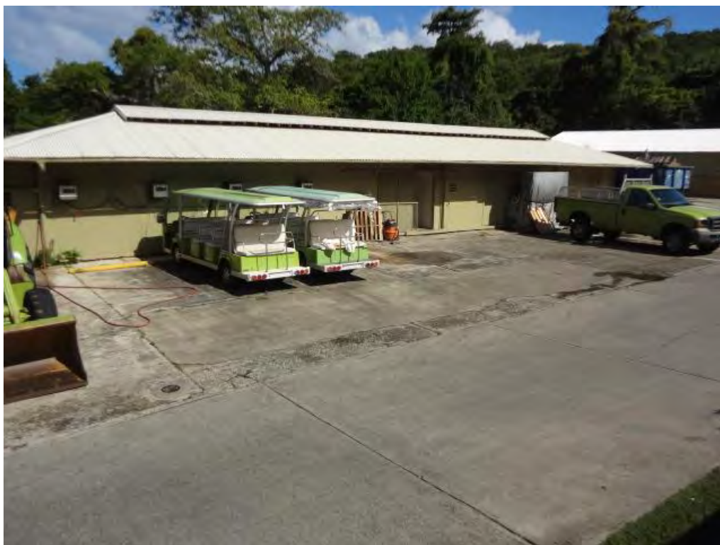
Former UST Location in Engineering Area
