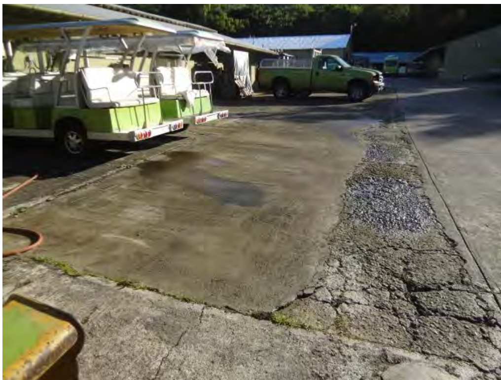
Concrete Pavement Patch at Former UST Location
