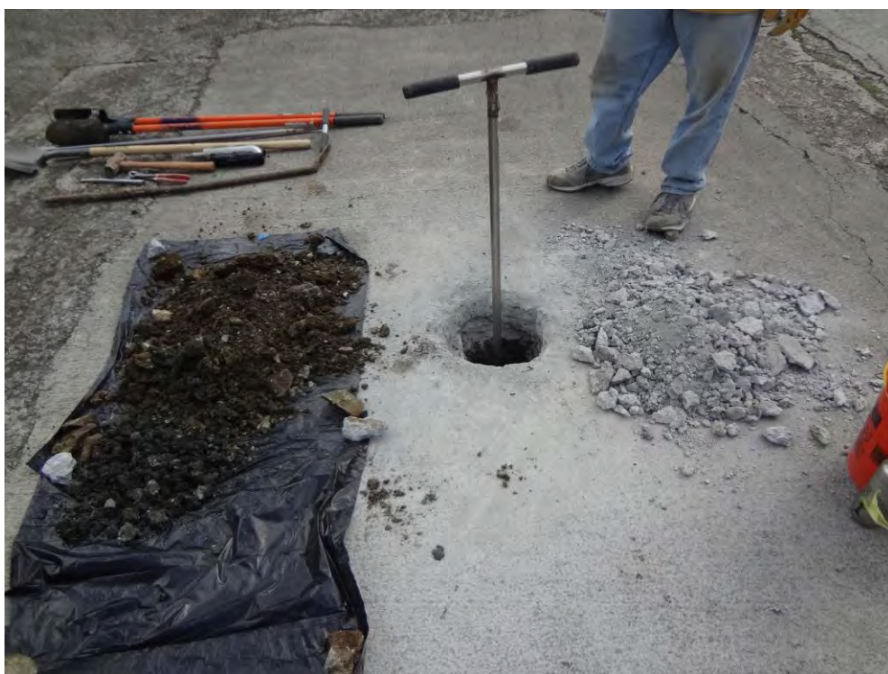
Former UST Location - Installing Borehole BH2
