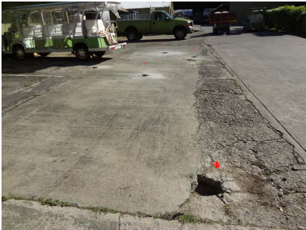
Boreholes Installed Through Pavement at Former UST Location – Borehole BH1 in Foreground
