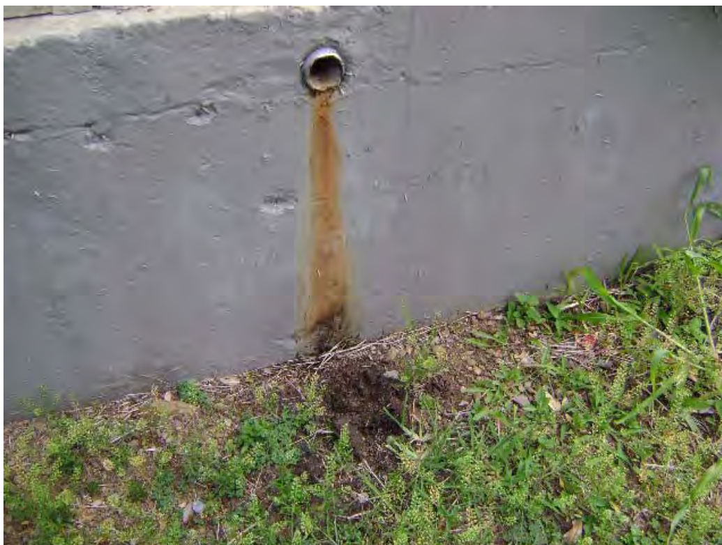
Oil Discharge From Floor of Emergency Generator Building to Soil Outside Building
