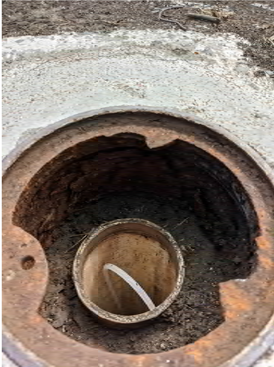
Photograph 13. View of surface completion of existing monitoring well MW-1. The vault and well screen/riser are perforated to the ground surface. Well may receive surface runoff from surrounding paved area.
