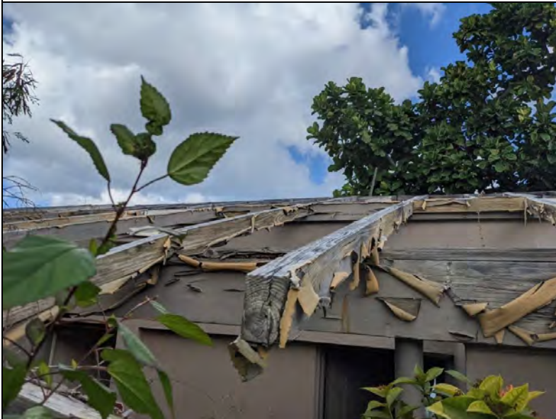
6. Roof and paint damage at Rooms 101 and 102 at Turtle Bay Estate.
