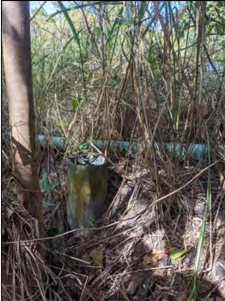
4. Possible asbestos-cement pipe identified in the northeastern corner of IA-2-01.
