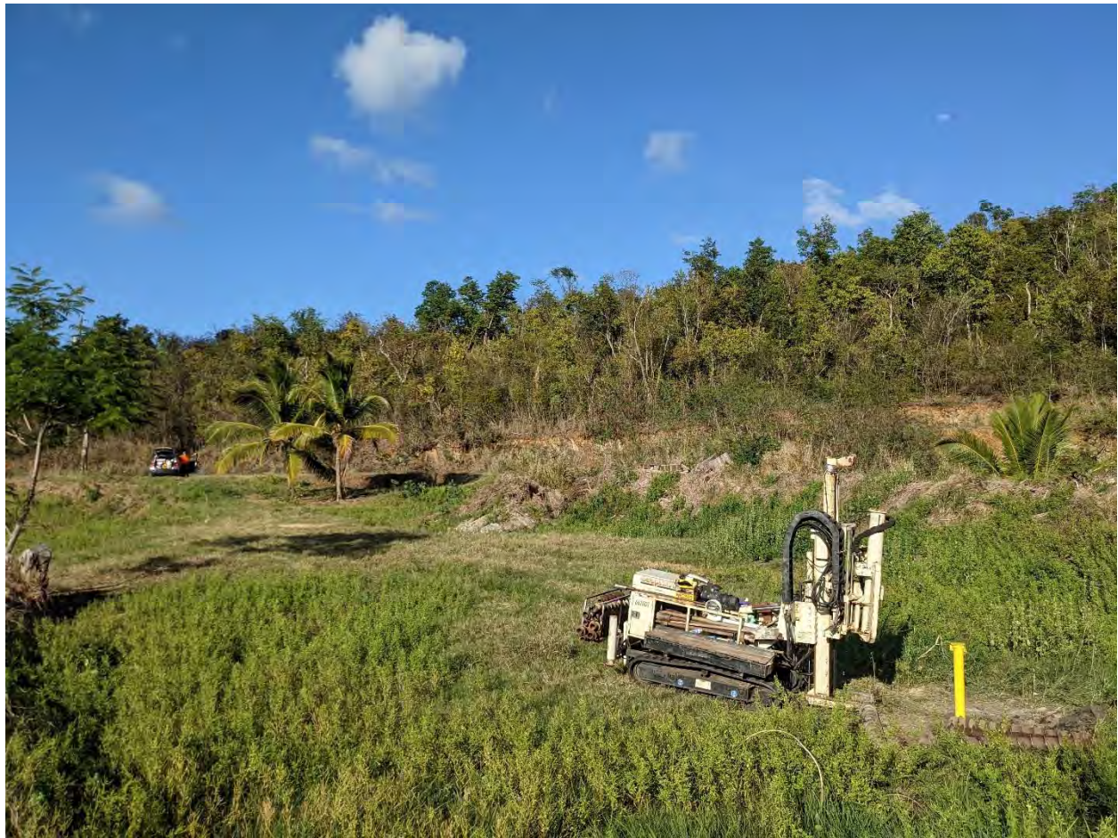
Photograph 10. View to north of monitoring well MW-3-01 installed at the southeastern edge of the debris landfill. VHB selected the well location to coincide with the locations of the apparent seeps observed along the southern edge of the landfill.
