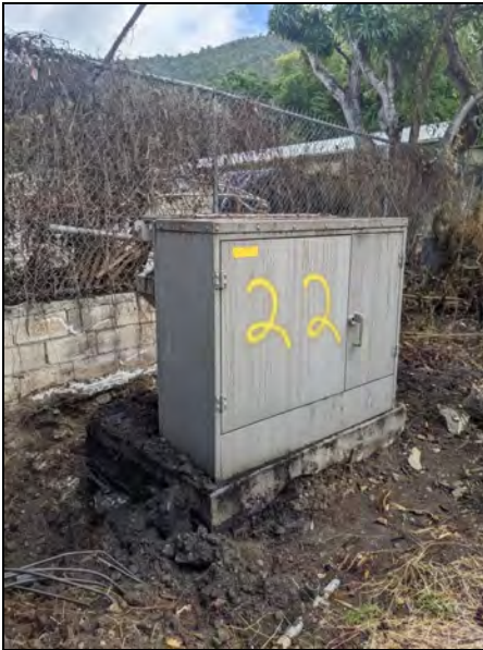
Leaking transformer within IA-2-02. Soil has been cleared away from transformer.
