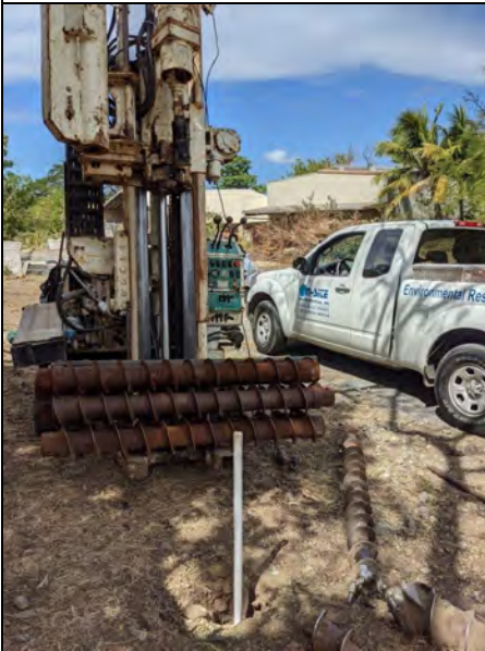
2. View of temporary piezometer installed at proposed MW-2-03 location.
