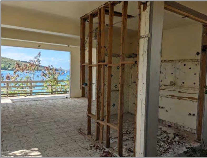
5. Partial demolition of Cottage Point rooms. Note removed tile and drywall and masonry, plaster, drywall, rubble with possible ACM.
