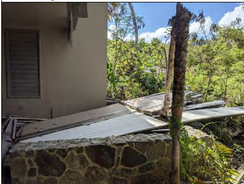
8. View to east of Hawksnest Beach rooms. Roofing debris, with roll tar paper with visible fibers, from different building (possibly Scott Beach ~500 feet to the east) visible in foreground.
