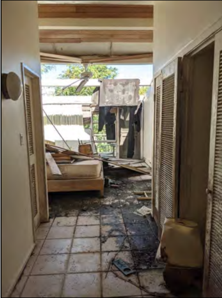
1. View of damage to second floor room at rooms 143-152. Roll tar paper with visible fibers behind.
