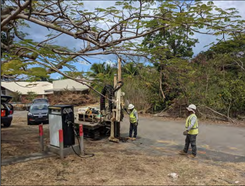
1. Drill rig set up at boring location SC-2-05, to the north of the ASTs and fuel dispenser.
