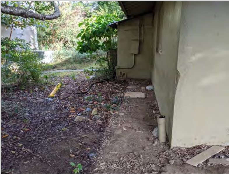
4-inch standpipe at corner of building in Area 2, identified by Fred Ianazzi as possible asbestos.
