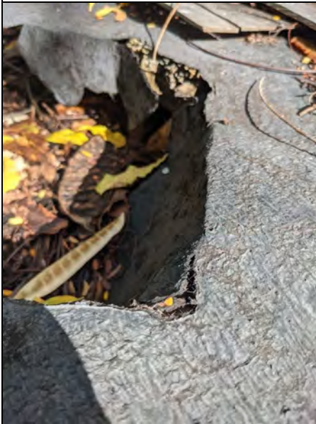
4. Roofing debris, including roll tar paper with visible fibers in Turtle Bay Estate courtyard.
