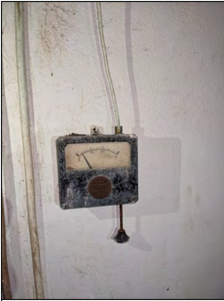
View of level gauge mounted on northern wall of Cottage 7 basement/bomb shelter. Medallion reads "The Liquidometer Corporation, Midget Levelometer. Serial 11." Based on the gauge graduations, the tank may have been ~ 300 gallons.
