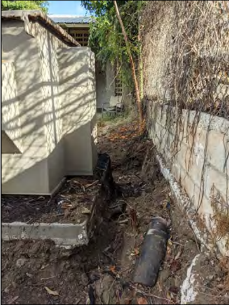
1. View behind leaking Transformer 22, in IA-2-02. Possible broken asbestos pipe in excavation.
