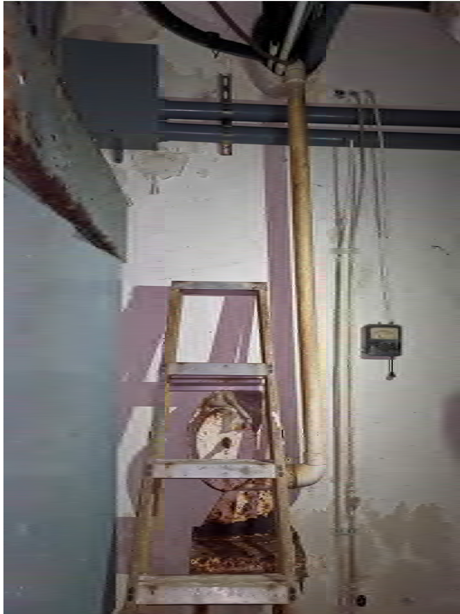
Photograph 4. View of tank level gauge and suspected metallic fuel lines observed in the basement at Cottage 7 (identified as the former bomb shelter by CBIA representatives). Metallic lines were traced to the exterior of the building using EMI.
