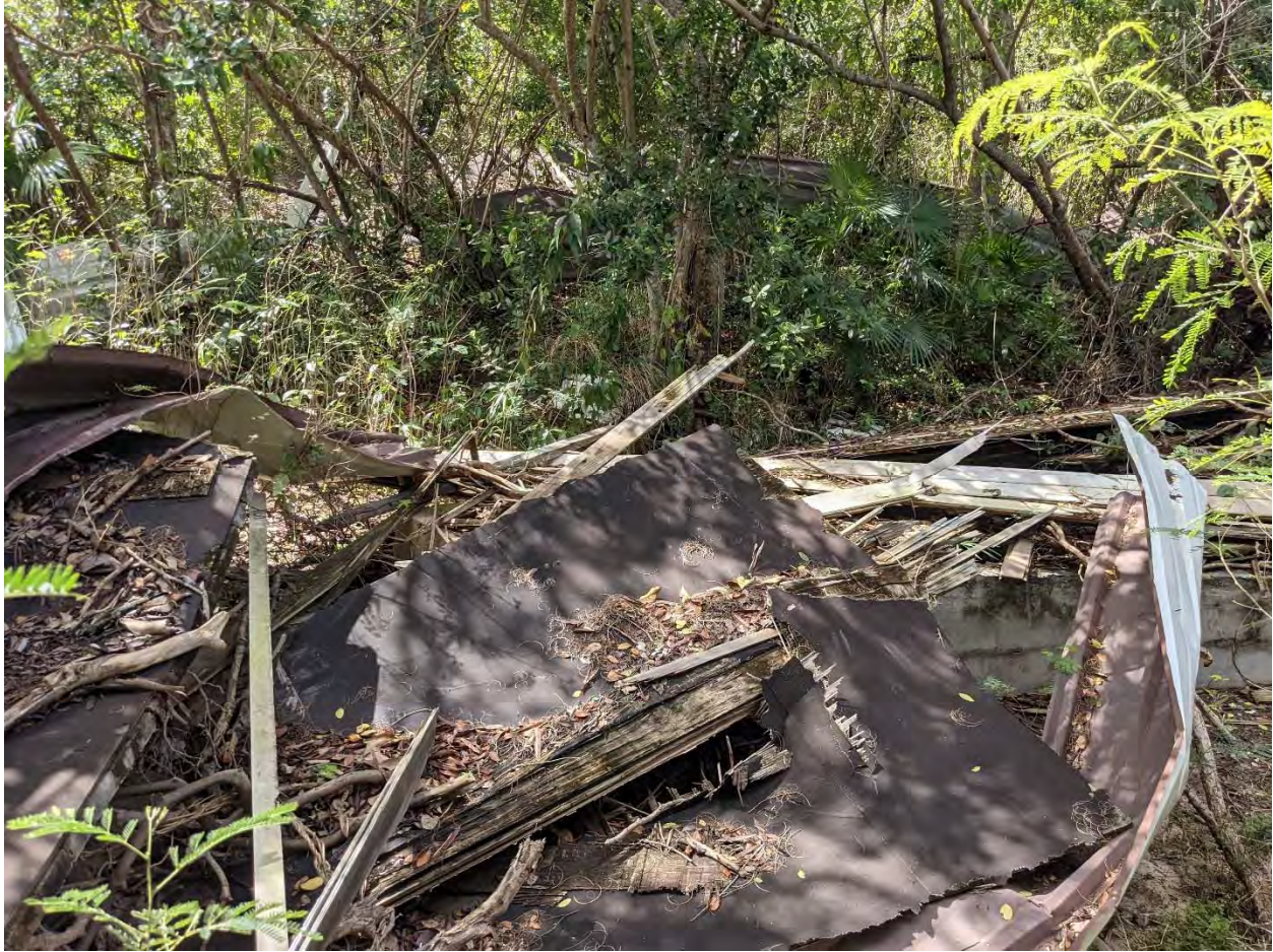
Photograph 2. View of roofing debris typical of that observed scattered across Site. Debris includes wood, sheet metal, and damaged tar paper with visible exposed fibers (possibly asbestos).
