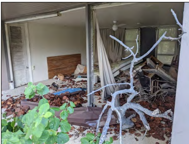
7. View through east side of first floor room at Hawksnest Beach. >1 foot of sand in room.
