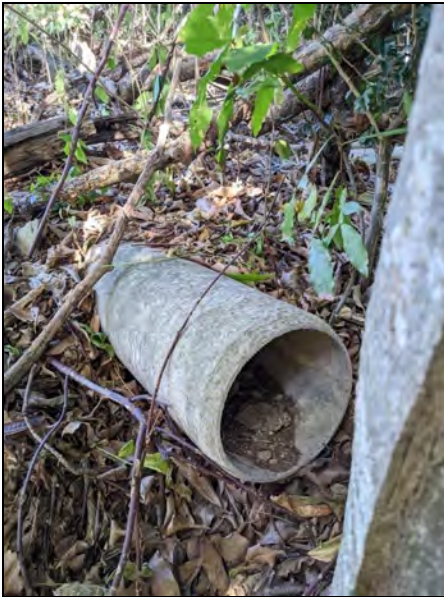
7. Possible asbestos pipe at the southern end of the gravel staging area
