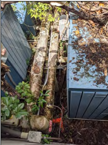
View of traced possible fuel line to area AC units and probable sanitary sewer manhole. Signal was lost beneath the AC units. GPR tracing of surrounding cleared areas did not locate any anomalies. GPR search was limited by debris, AC units, and dense vegetation.
