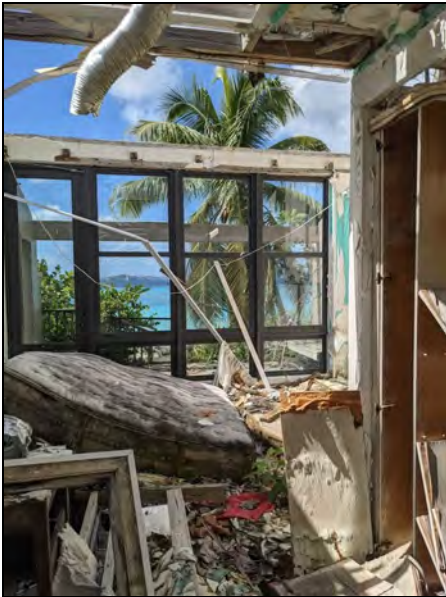
9. View of damage to Scott Beach rooms - view through room to west. Note missing roof and missing/damaged sheetrock/plaster ceiling.
