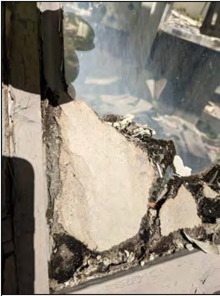
9. View of drywall debris with visible fibers in southern Caneel Beach room.
