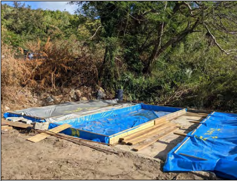
11. View looking south of apparent containment pads built on former WWTP pump house concrete pad. Tarps are labeled with "Tran. #22" and "Tran. #23".
