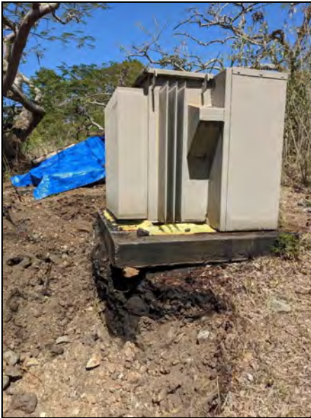
3. View of leaking transformer 23 near Sugar Mill Ruins. Note soil pile behind. Note concrete is wet with oil, sorbent pads are saturated; transformer appears to be continuing to leak.
