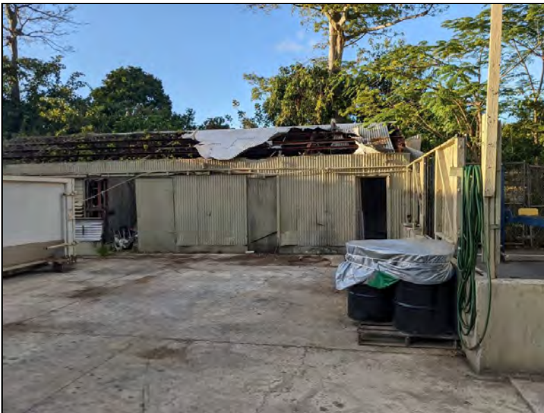
3. IDW drums (2 soil, 1 water) placed on a pallet, covered, and stored in the engineering area.
