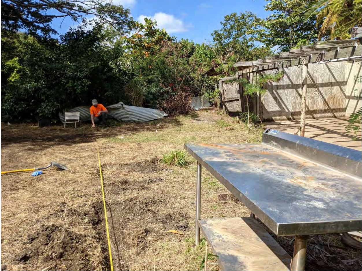
Photograph 5. View of asbestos pipe identified during the Level 2 investigation in Area 2 located and exposed. Pipe appears to head to the west towards the former greenhouses. Similar, possible asbestos pipes were observed in other areas of Area 2 and in Areas 1 and 3. Debris in background limited access to parts of IA-2-04.
