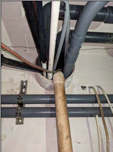
View of pipes leaving northern wall of Cottage 7 bomb shelter electrical room through possible asbestos carrier pipe. Note level gauge and possible fuel lines to right.
