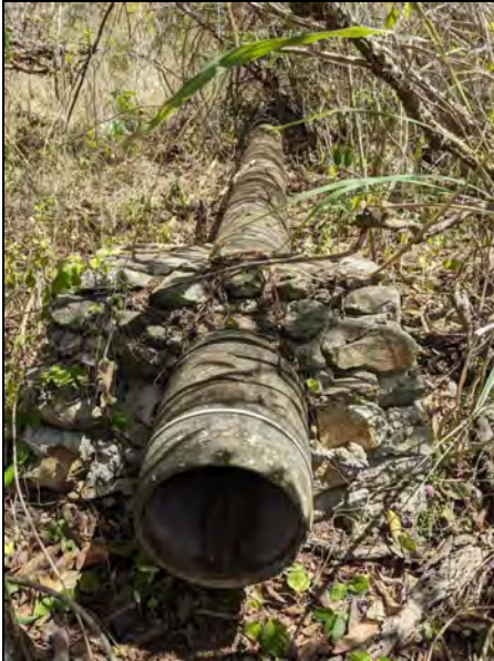
4. Possible asbestos-cement pipe north of landfill access road.
