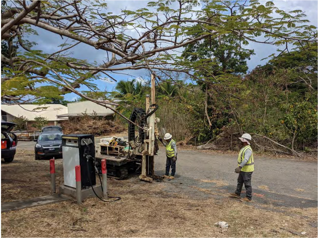
Photograph 12. View of subsurface soil sampling at SC-2-05, immediately to the north of the fuel dispenser. VHB observed visual, olfactory, and PID evidence of petroleum contamination in the soil core at this location from approximately 3.5 to near refusal at 23 ft bgs.
