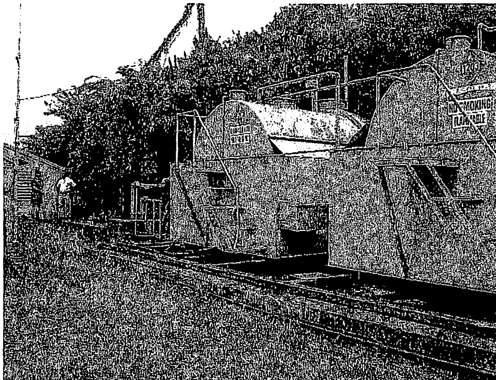
Above Ground Fuel Storage Tanks at Marina Facility
