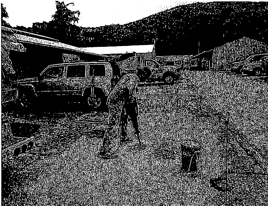
Former UST Location - Cutting Pavement for Borehole BH2
