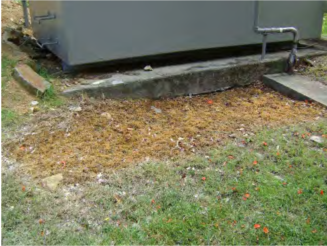
Distressed Vegetation & Fuel Impacted Soil Near Gasoline Fuel Tank North of Generator Building
