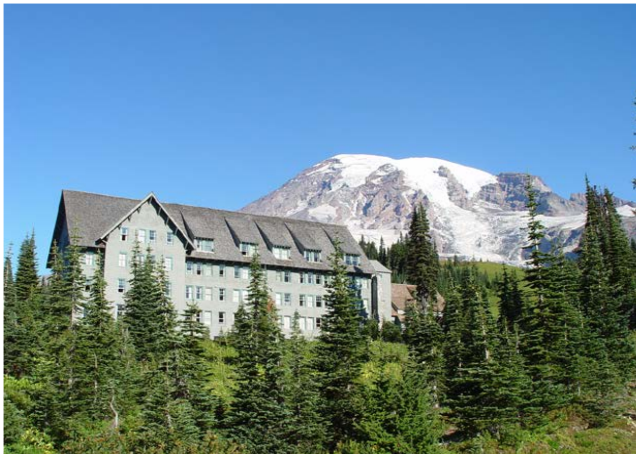
Figure 4. Paradise Inn Annex Photo Source: Kirk Associates, 2011.
