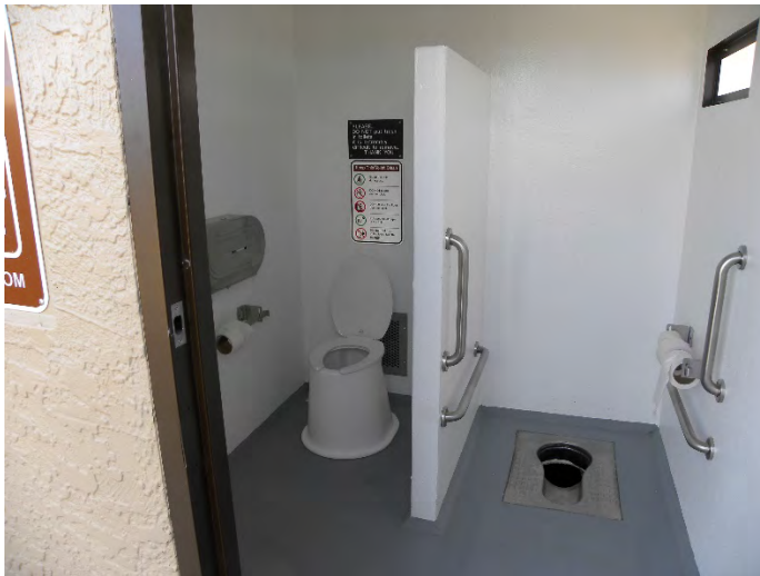
Figure 3.71 Squat toilet adjacent to a standard toilet riser allows users with different preferences to have options. Photo provided by CXT.
