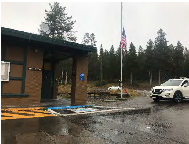
Figure 3.14 Striping in many different colors is visually unattractive and requires more maintenance.
