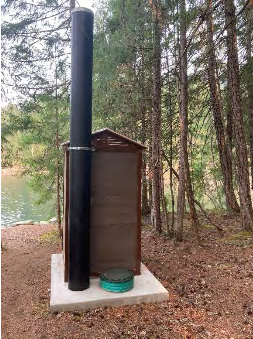
Figure 3.78 North Cascades National Park, Ross Lake Campground vault toilet cleanout. Make sure that the backside of the vault toilet is easy for a pumper truck or in this situation a pumper barge, to access. Materials. Make prefabricated vault toilet buildings out of concrete or masonry. If located in a very hot climate, insulate the roof to ensure the proper air currents and functioning of vault ventilation.
