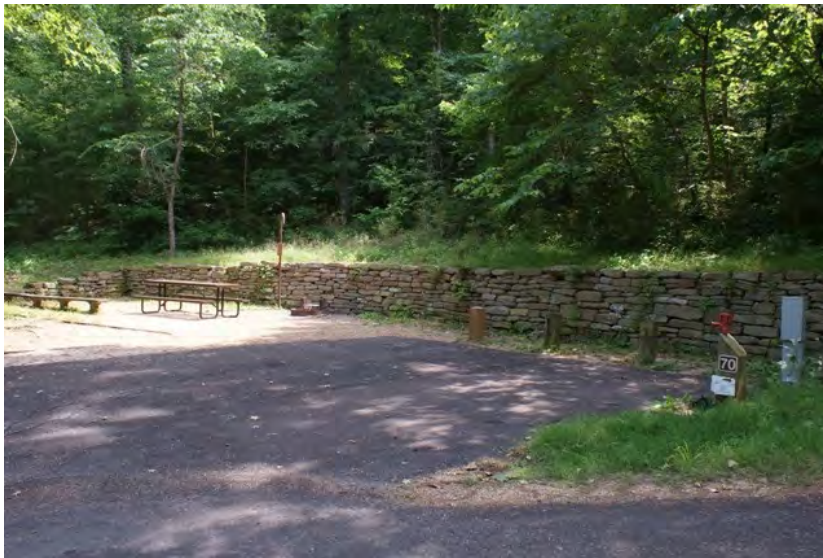
Figure 3.42 Buffalo National River, Arkansas, Buffalo Point Campground stone retaining wall.
