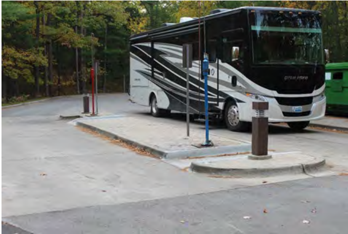
Figure 3.106 Platte River campground dump station includes an accessible RV parking lane with island access aisle to approach station components (Sleeping Bear Dunes National Lakeshore).
