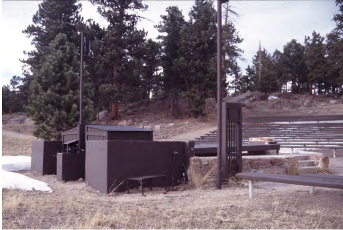
Figure 3.90 A “before image” of Moraine Park Amphitheater. The amphitheater was developed in the 1950s, had out-of-date technology and in-accessible seating areas. (Rocky Mountain National Park)
