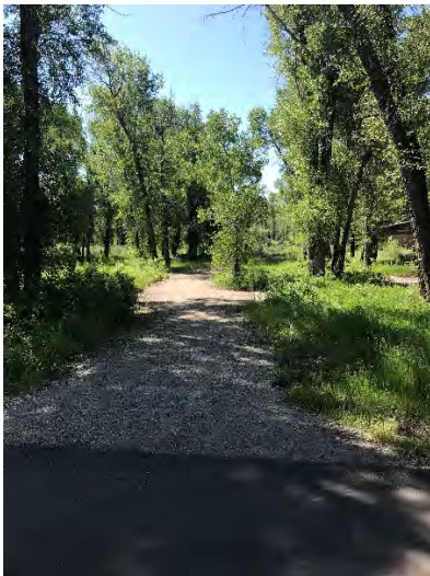
Figure 3.43 Six-foot-wide accessible crusher fine aggregate trail to comfort station. (Crusher fines can be accessible if compaction and slope requirements are maintained.)
