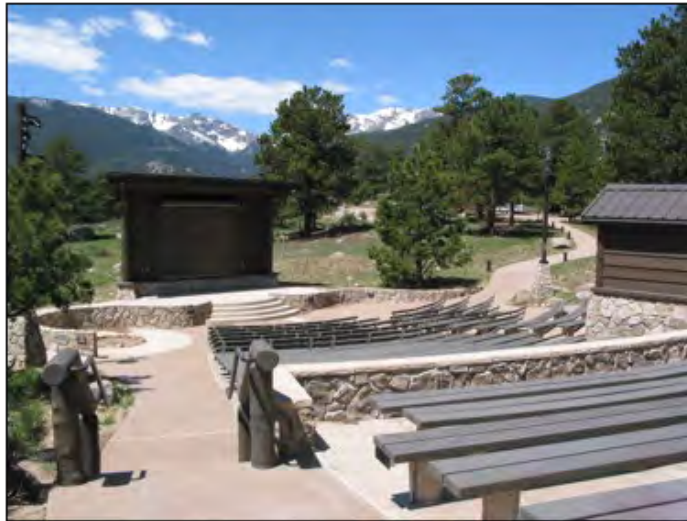
Figure 3.91 The “after” image of the same amphitheater updated technology and provides accessibility to 50% of seating, including 10 wheelchair spaces integrated throughout. Seating includes benches with and without backs to enhance comfort and usability for all visitors. (Rocky Mountain National Park)
