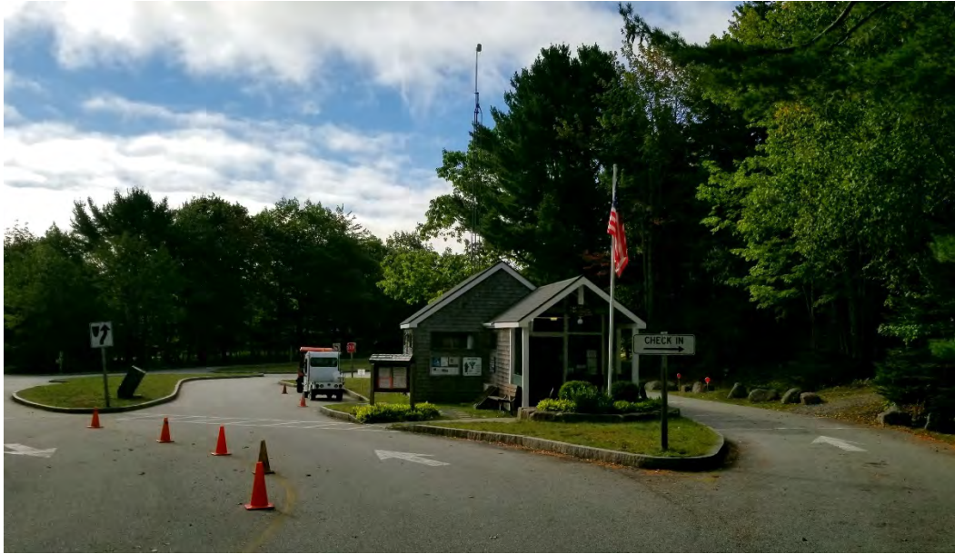
Figure 3.2 The Blackwoods Campground check-in area with a building that represents the park architectural vernacular.
