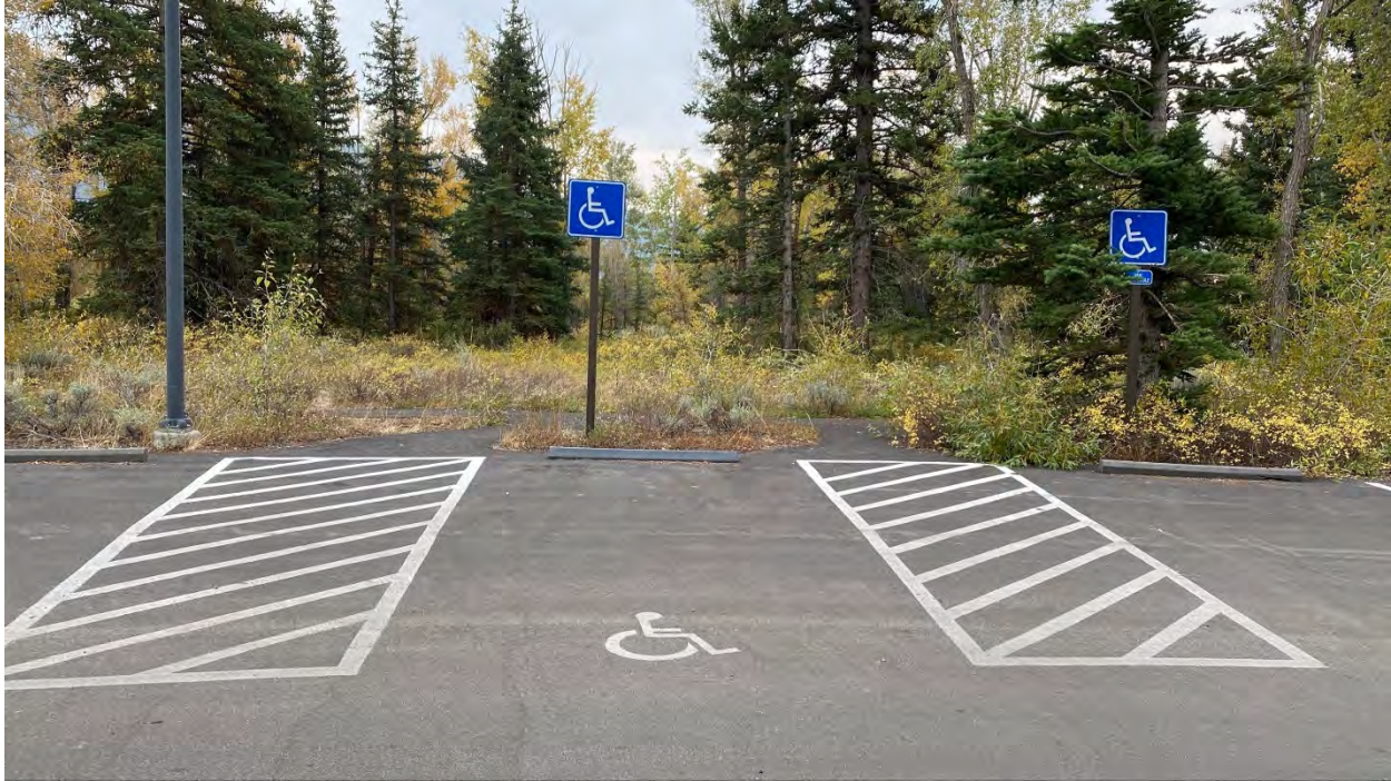
Figure 3.15 Accessible parking space with white parking and white aisle.
