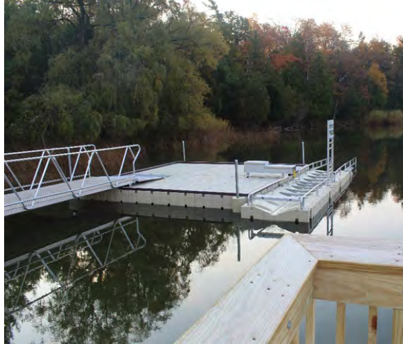
Figure 3.54 An accessible kayak/canoe launch provides a wheelchair transfer bench, rails to assist getting in and out of the watercraft, and water level adjustment. (Loon Lake at Sleeping Bear Dunes National Lakeshore).
