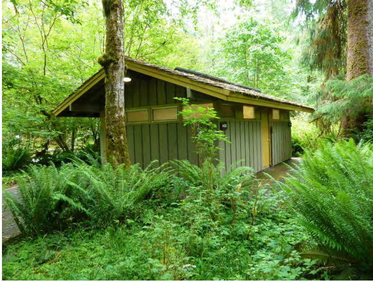
Figure 3.74 Prefabricated toilets can be ordered in a variety of styles in effort to meet the park architectural character. To soften the appearance of newly installed vault toilet units, revegetate with native plants. (Hoh Rainforest, Olympic National Park).
