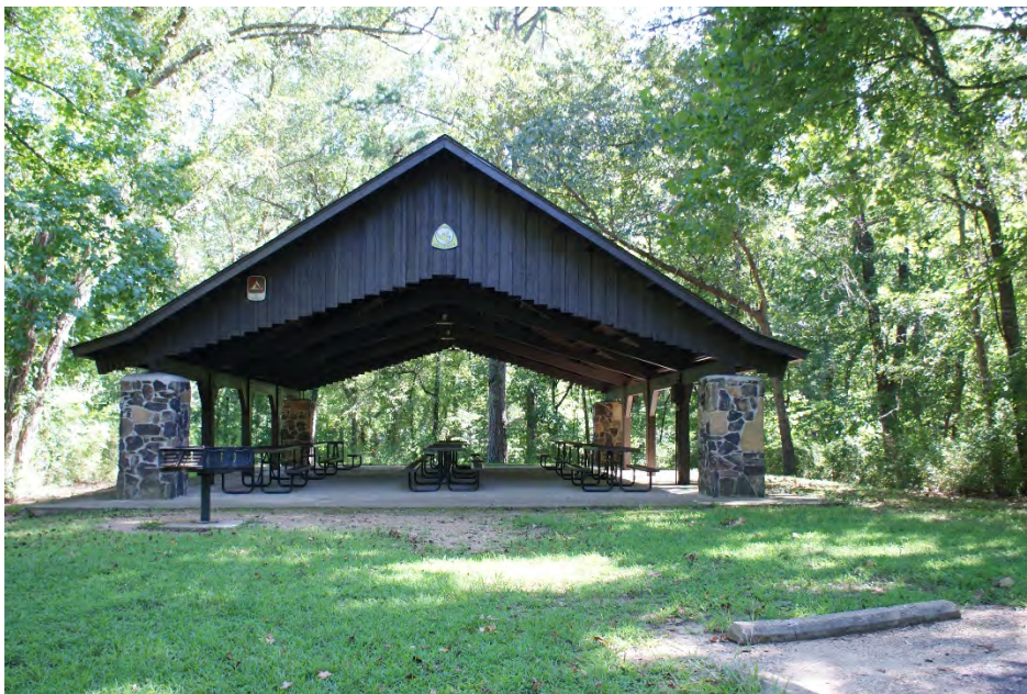
Figure 3.96 Picnic pavilion at Buffalo National River, Arkansas, Buffalo Point Campground.
