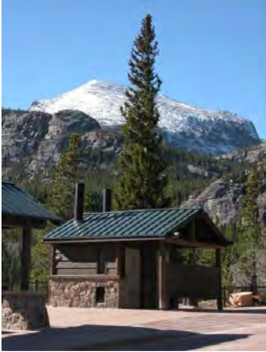
Figure 3.73 This custom built vault toilet at Rocky Mountain National Park uses durable materials and aligns with the park's character. Siting vault toilets so that the stacks are high and south or west facing is critical for sweet smelling toilets.
