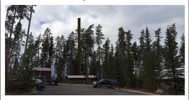
New 80' Unipole Tower with Interior Antennas and Equipment Shelter
