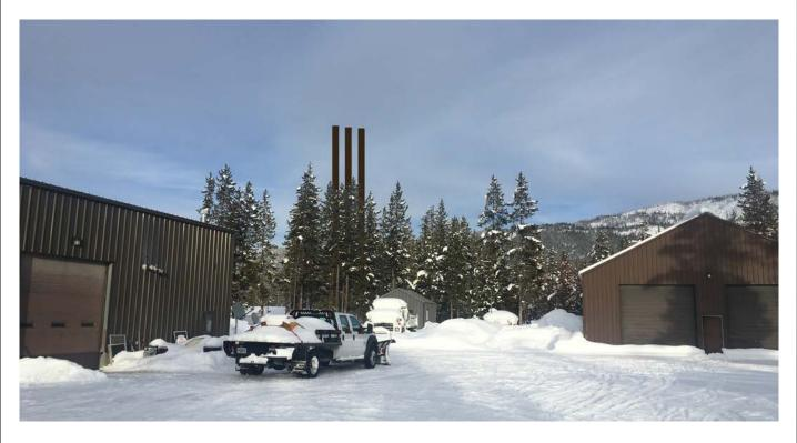
(3) New 80' Unipole Towers with Interior Antennas and Equipment Shelter
