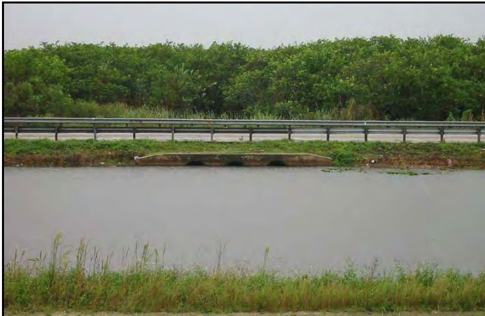
Figure 3-21 – One of 19 Sets of Existing Culverts (Facing South from L-29 Levee)
