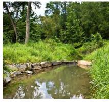
**Figure 5-5.** Rock revetment structures provide durable protection to the lower portion of the streambank, and may be combined with integrated bank treatment (source: James Long Park, Prince William County Environmental Services).
