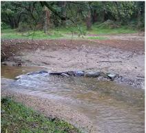
**Figure 5-8.** J-hook vanes direct erosional forces away from unstable streambanks and improve aquatic habitat by forming scour pools (source: Montgomery County, MD "Stream Restoration Techniques").
