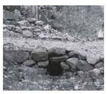
Figure 5-33. Rock trail culvert (USFS).
