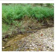
**Figure 5-3.** Branch layering stabilizes the bank with alternating layers of soil and live branches. Branches extend from the stabilized face of the bank into the original bank material (source: Montgomery County, MD, "Stream Restoration Techniques").
