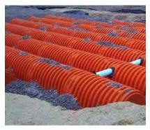
**Figure 5-16.** Sub-grade retention system (StormChambers).
