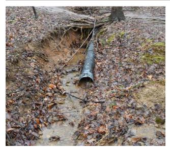
**Figure 3-167.** Slope washout near east boundary (QE, 2020).
