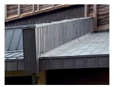
**Figure 5-53.** Standing metal seam roof, Filene Center (QE, 2020).
