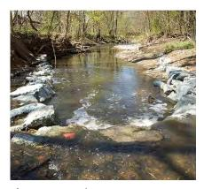
**Figure 5-7.** Rock cross vanes are constructed to provide grade control and reduce bank erosion (source: Montgomery County, MD "Stream Restoration Techniques").
