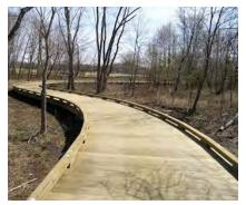
**Figure 5-36.** Curved boardwalk with curb (Boardwalk Design Company).
