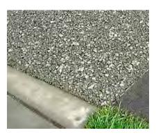
**Figure 5-15.** Permeable concrete (The Concrete Network).
