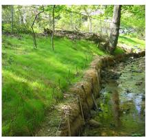
**Figure 5-2.** Fiber rolls are made of coconut fibers bundled together with biodegradable netting, and can provide temporary protection for the bank while vegetation is established (source: Montgomery County, MD "Stream Restoration Techniques").
