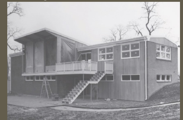
Existing clubhouse under construction, 1964.
