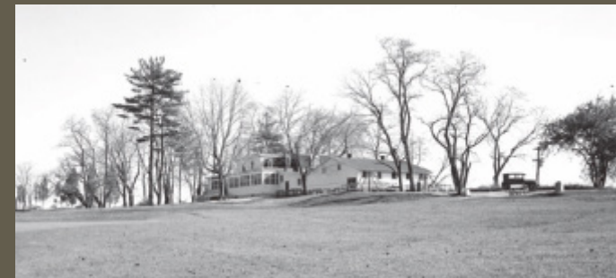
Farmhouse on site that was used as the golf clubhouse from 1923-1964.
