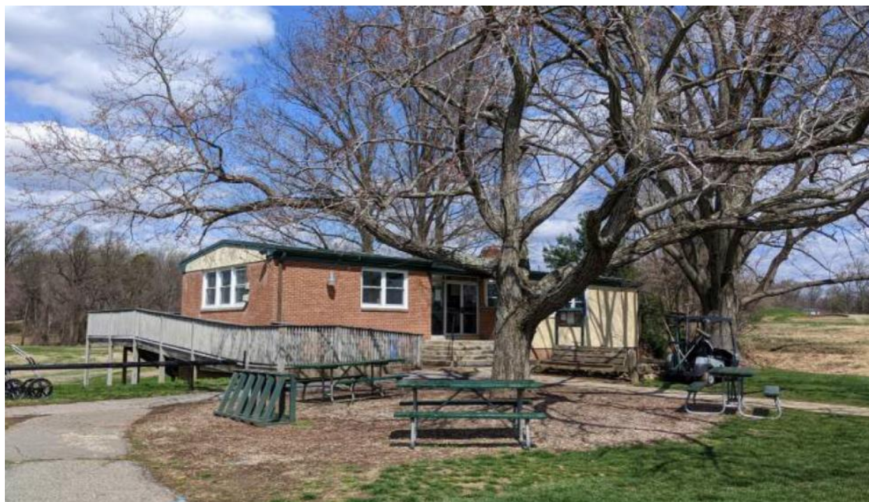
View of the front and southwest side of the Mission 66-era clubhouse
