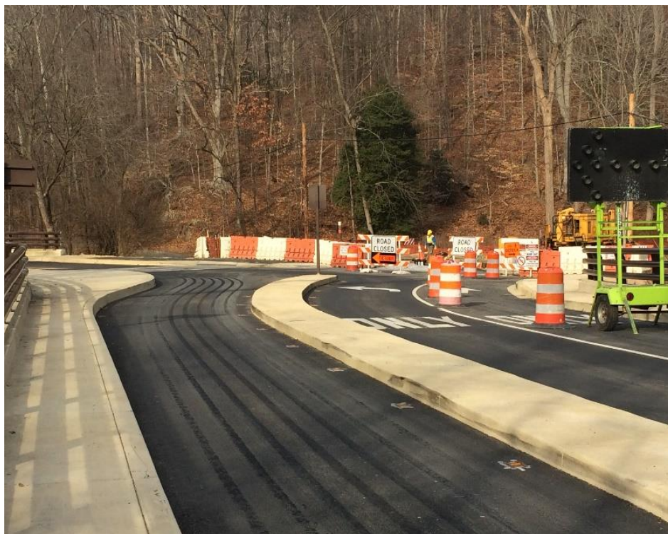
Beach Drive NW reconstruction project
