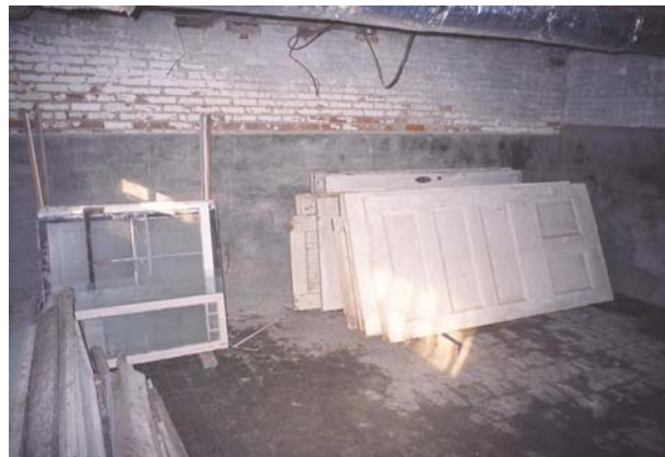
Figure C - 16 Original doors in storage in Room 001
