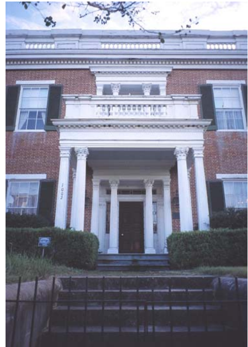
Figure B - 2 Front view of the adjacent Balfour House; it is likely the Willis-Cowan House originally had a similar front porch
