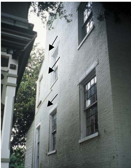
Figure C – 1 Stack joint on east elevation
