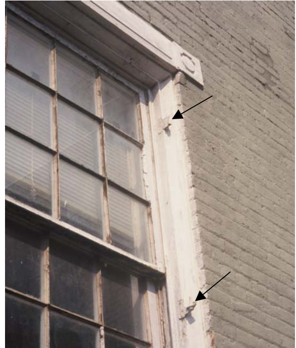
Figure C – 10 Shutter hinges; the upper hinge dating from the second quarter of the nineteenth century, the lower dating from the third or fourth quarter or the nineteenth century
