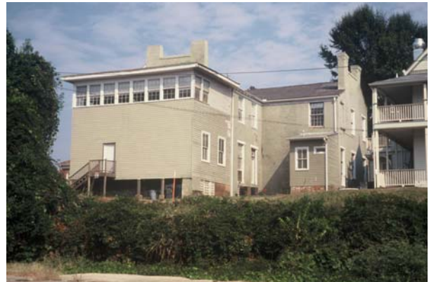
Figure B - 6 Southeast oblique of the house showing two-story frame portion with sleeping porch on second floor
