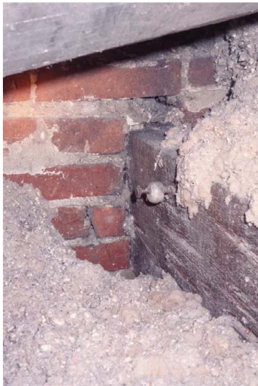
Figure B - 3 Ceiling joists above the original L-shaped porch are resting in formed joist pockets in the brick wall, indicating they are an original feature
