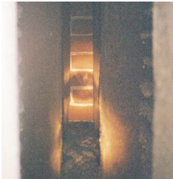
Figure C – 7 Pencilled brickwork visible in pocket door opening to Room 206A
