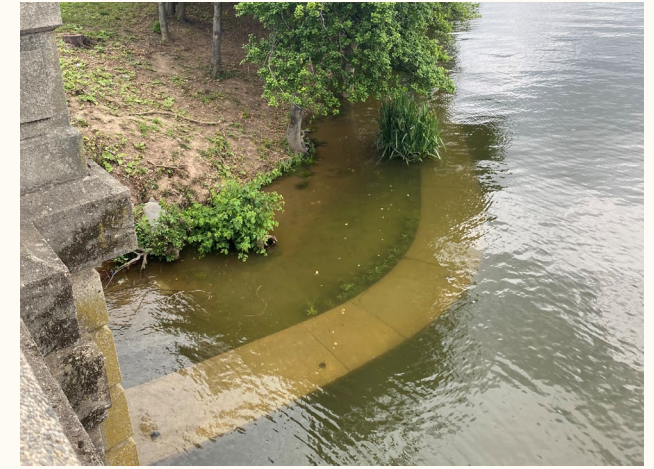
Tidal Basin West – Looking North from Inlet Bridge
