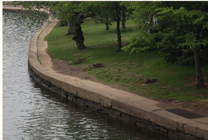
Tidal Basin East – Looking East from Inlet Bridge
