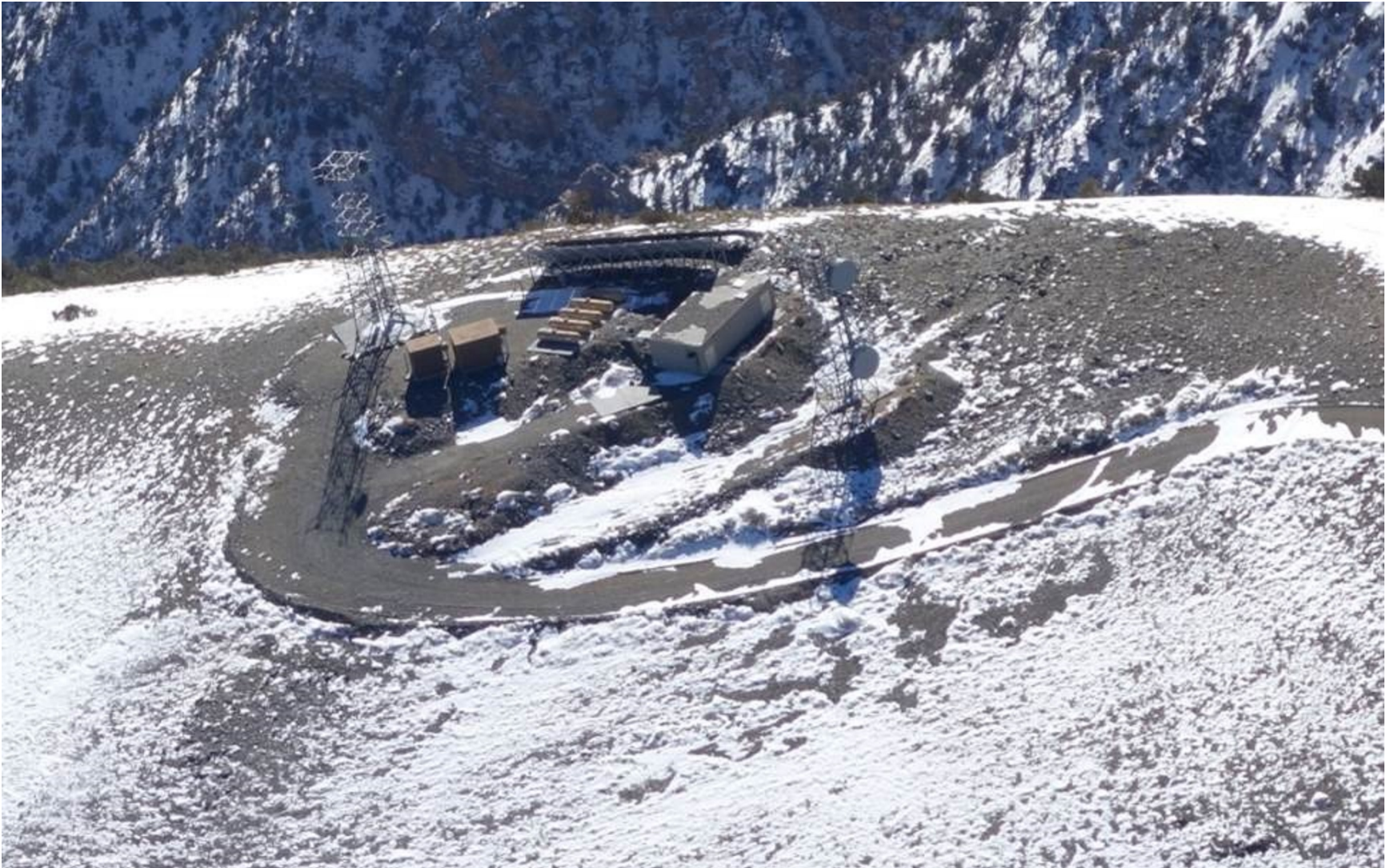
FROM LEFT TO RIGHT: US AIR FORCE TOWER, NPS COMMUNICATIONS BUILDING, US AIR FORCE COMMUNICATIONS BUILDING, FUEL DEPOT, SOLAR PHOTOVOLTAIC ARRAYS, CALTRANS COMMUNICATIONS BUILDING, CALTRANS TOWER. REMOTE AUTOMATED WEATHER STATION NOT SHOWN.
