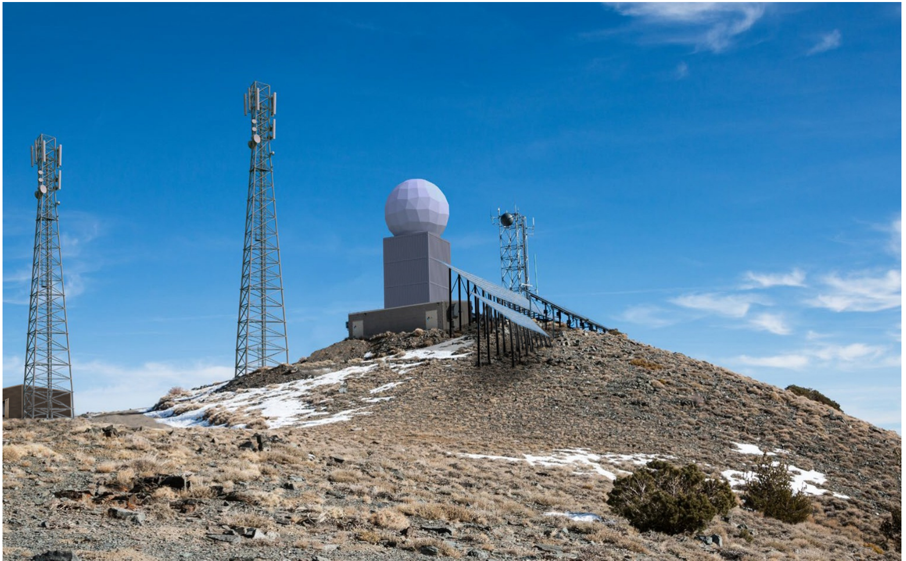
FROM LEFT TO RIGHT: PROPOSED AT&T COMMUNICATIONS BUILDING, AT&T TOWER, CALTRANS TOWER, CALTRANS COMMUNICATION BUILDING, US NAVY RADOME, SOLAR PHOTOVOLTAIC ARRAYS, US AIR FORCE TOWER
