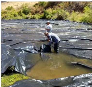
Black plastic treatment of upper slough at RM -12(NPS)
