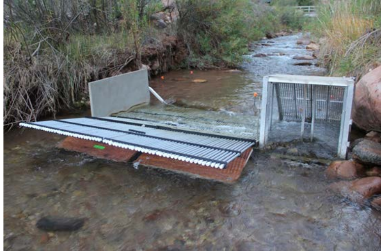
FIGURE 2-2. Example Weir at Bright Angel Creek to Intercept Spawning Non-Native Fish
