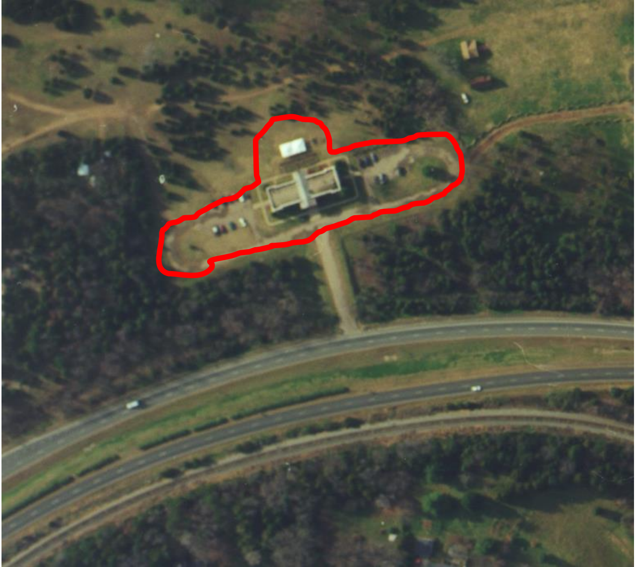
Figure 2. Visitor Center, Parking Lots, and Septic Field. (Looking West)
