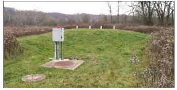
Figure 16. Example of a Mounded Sand Filter
