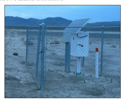
**Photograph 1.** Existing solar impressed current system with chain link fence perimeter.
