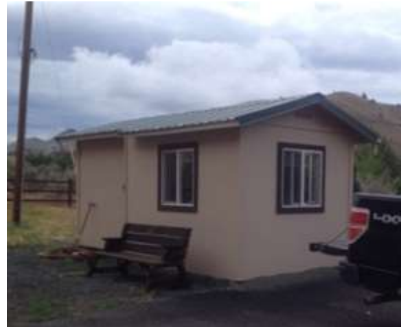
Figure 3: Water Treatment Building
