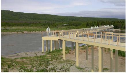
One conceptual design for the proposed river crossing is a short-span pile supported wood frame bridge (view to the north)
