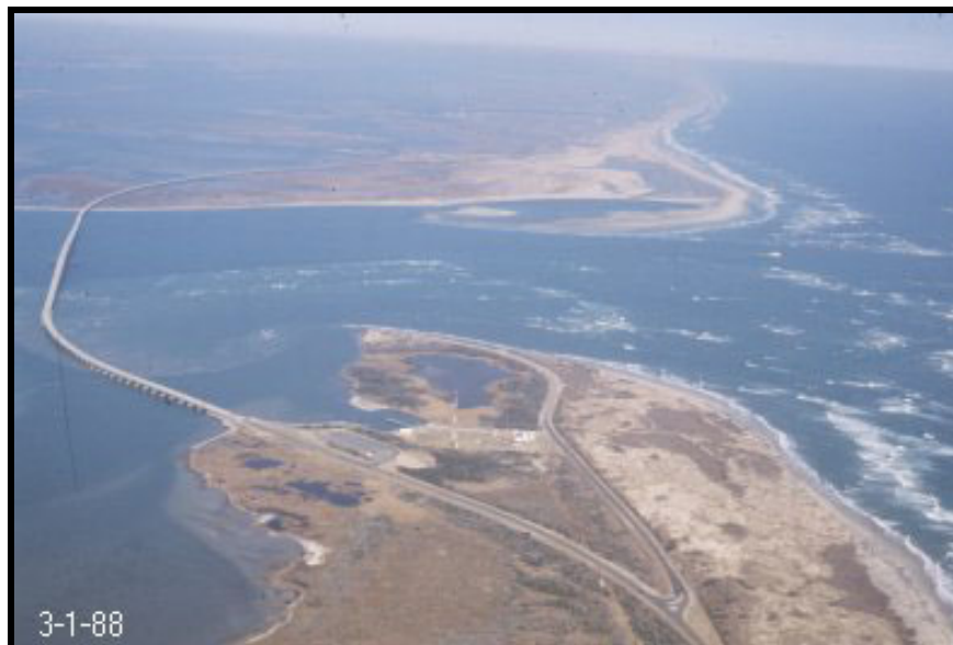
Figure 2-3. Looking north from Oregon Inlet to southern Bodie Island.
